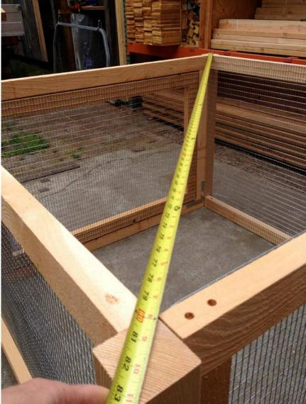
7. Next, make sure the run is level. If not, you can lift up the low side and place a thin paver or a stone until it is level across the top of all four frames.
