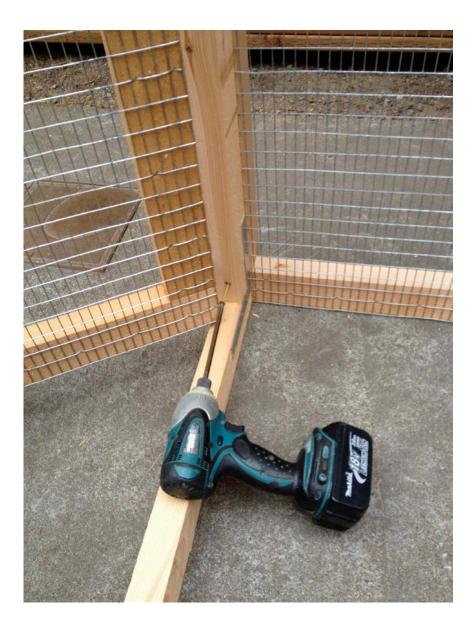
Now the square the assembled run by measuring the diagonals and adjusting until he two diagonal lengths are the same (should be about 83 5/15")
